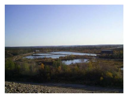
Fig. 8. Collection and polishing ponds at the Rabbit Lake Operation, Saskatchewan. Only water meeting applicable regulatory guidelines is discharged to the receiving environment.
