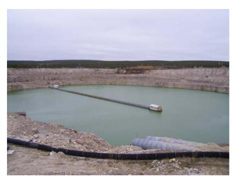
Fig. 7. In-pit tailings management facility (TMF) at McClean Lake. Water is pumped and circulated to ensure tailings consolidation at the pit bottom and designed water level is maintained in the pit lake.
